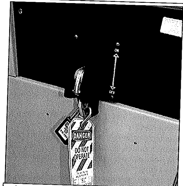
Electrical Power Lockout & Tagout
